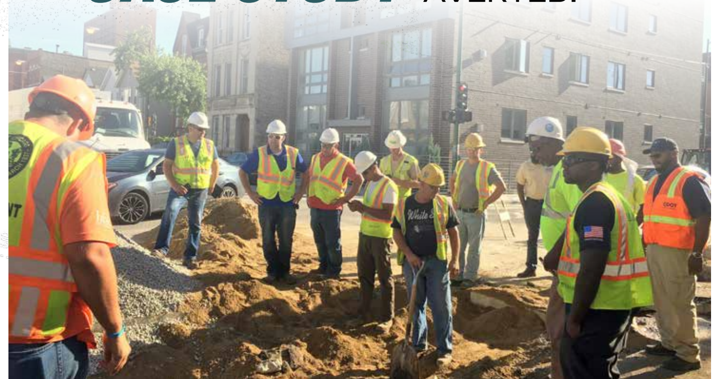
Left: Saw cutting to find the extent of a void beneath a Chicago city street. Above: Utility engineers on site.
