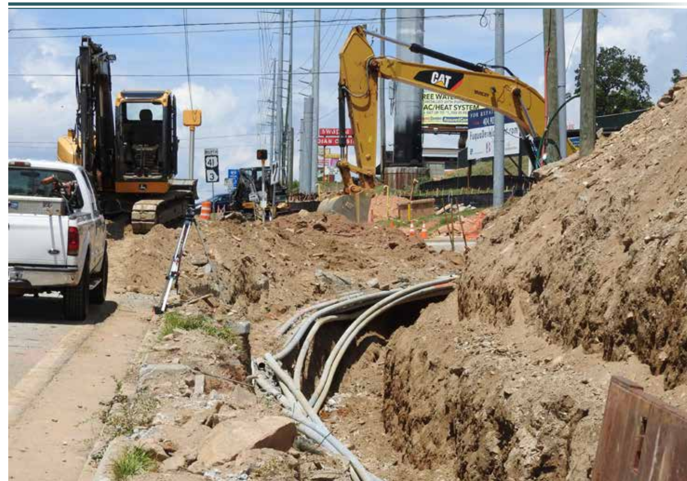
This photo was taken by me to compliment BRI Utility Construction. They are one of the two utility contractors that I have seen set up a surveyor's level so that they could check grade. BRI was adjusting a nine-way telephone ductbank that was situated in conflict with a storm drain that was proposed to drain US 41 at the recently constructed Atlanta Braves Stadium.
