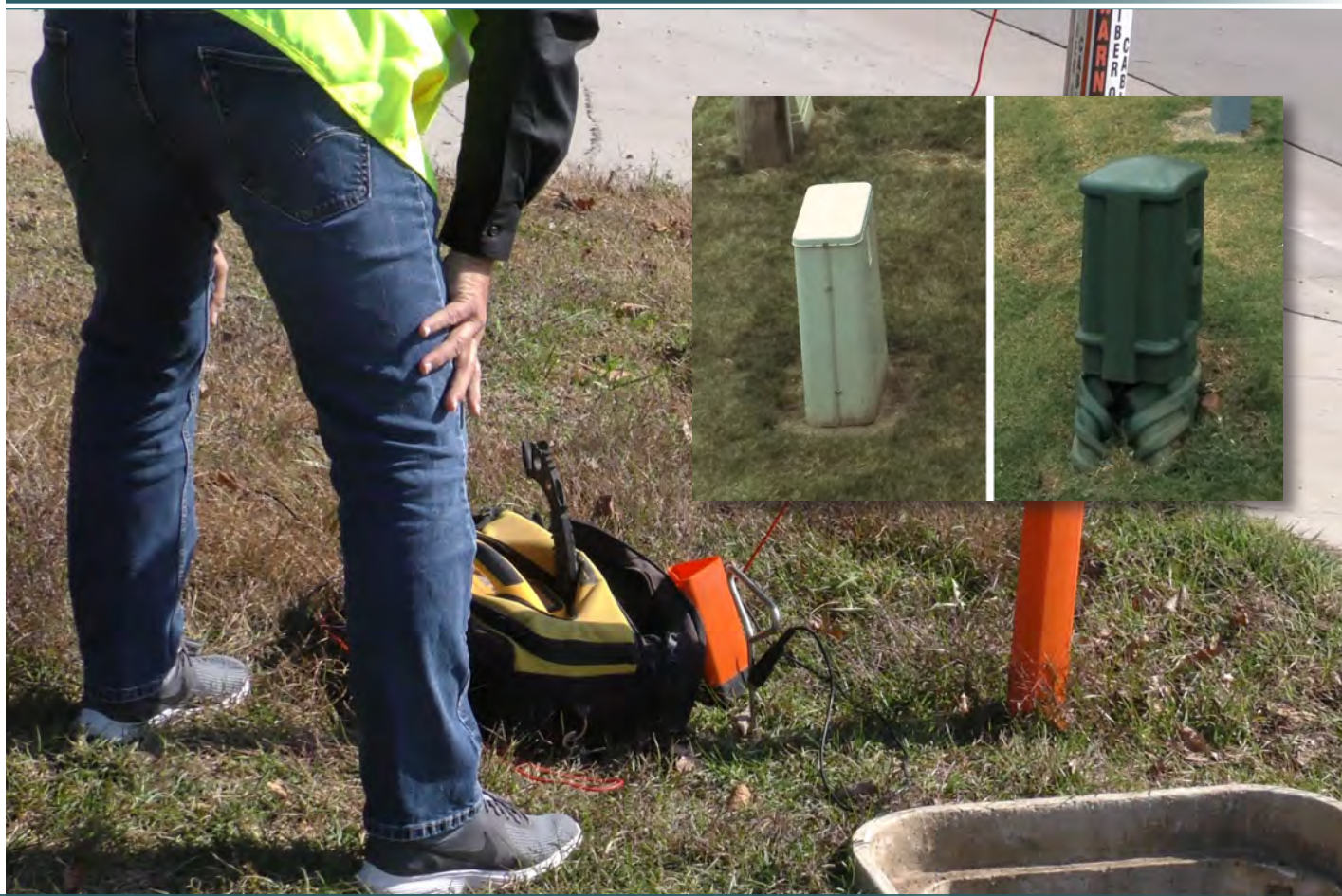
Top: Mike Parilac hooks up his transmitter to test the tracer wire viability on the job, which checks out ok. Top Right: These above ground telephone structures indicate the presence of parallel-positioned telephone duct. Bottom: The 4-foot ground rod (left) was used before being switched with a portable ground rod (right).
