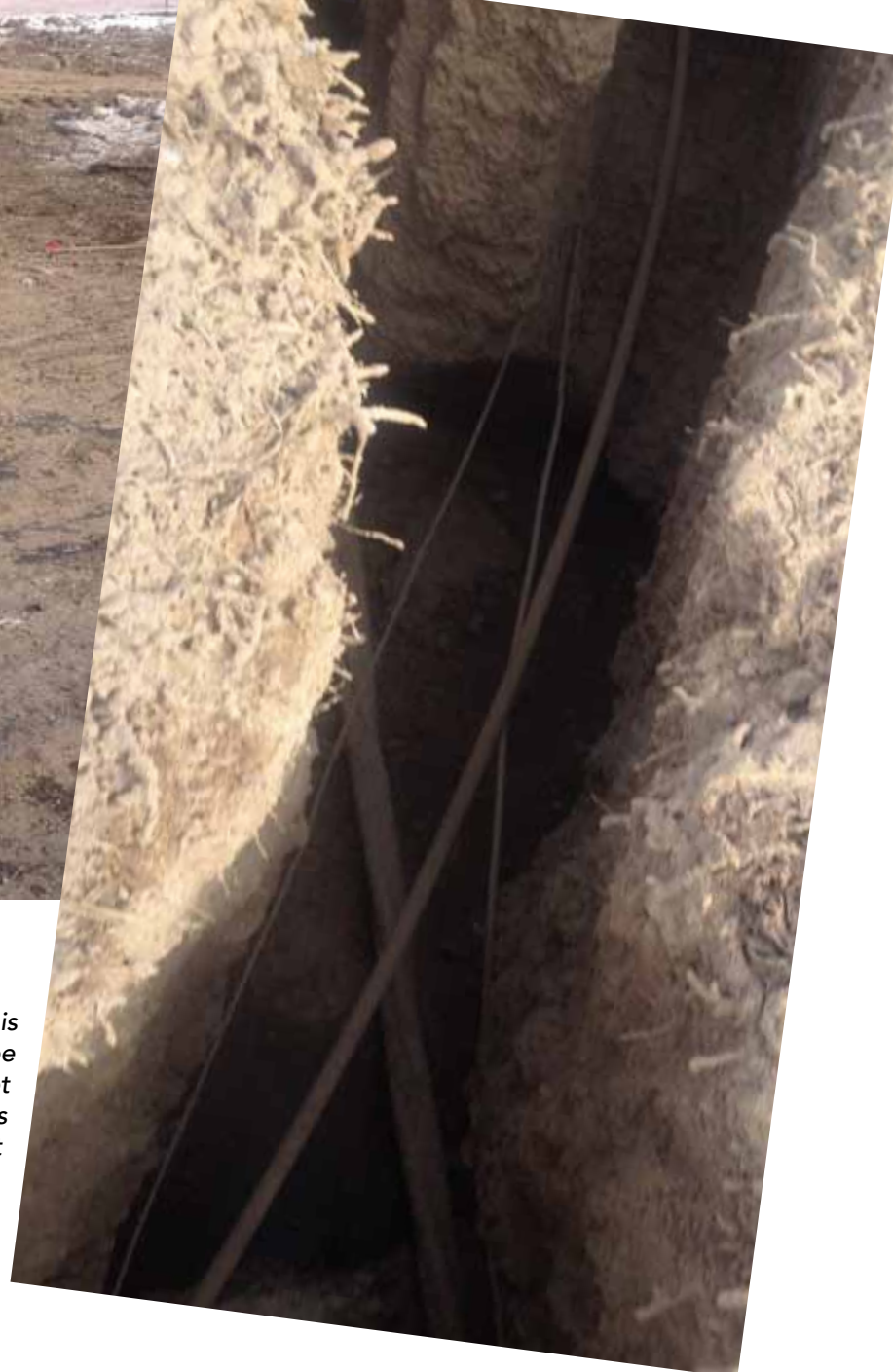
Exposing entire spans of buried cables in a right-of-way.
