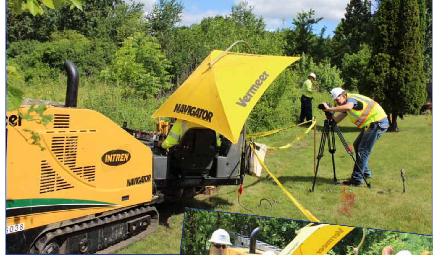
Above: Shooting footage of a horizontal directional drill in action.
