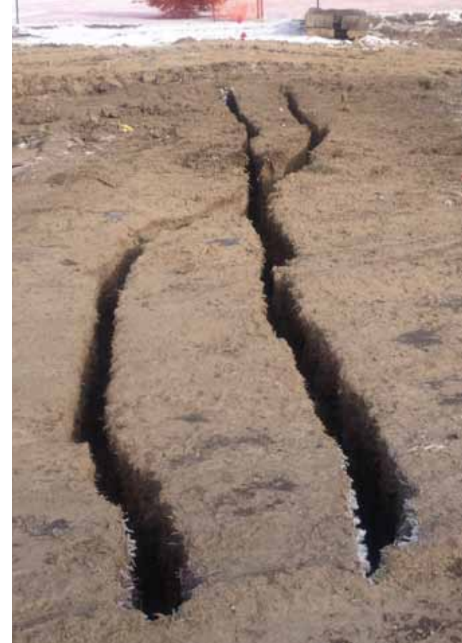
Exposing entire spans of buried cables in a right-of-way.
